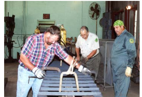
Employees lay out the metal to be welded on the ramp.
