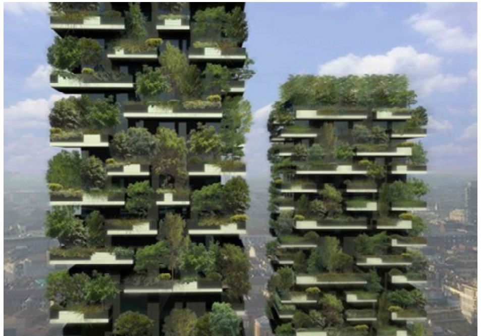
The biggest challenge was calculating the loads created by all that greenery blowing in the wind (Boeri Studio)
