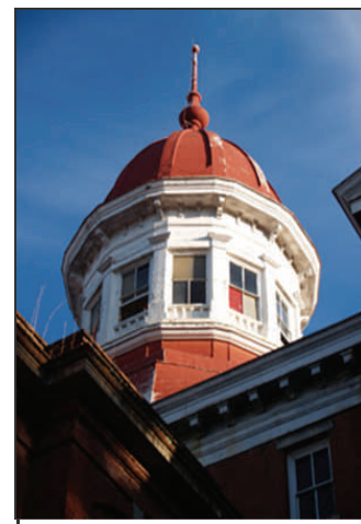
Babcock Building Cupola
