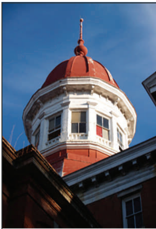
Babcock Building Cupola
